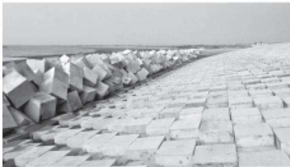
Figure 8.1: Revetment for the Maheshkhali Channel Shore Protection in Cox's Bazar
